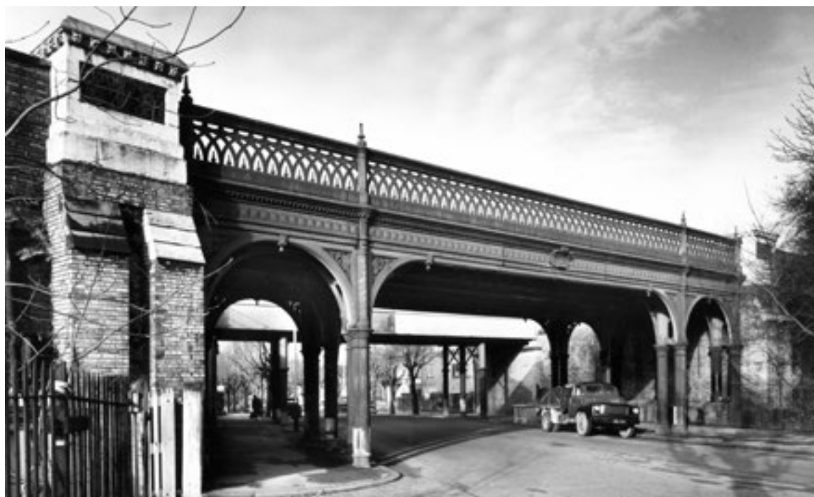
Rosendale Road bridge before removal of columns and the goods depot bridge behind, photo c1966
