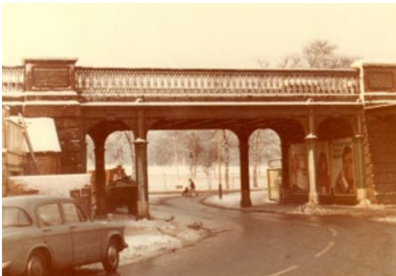
Croxted Road bridge, photo c1975
