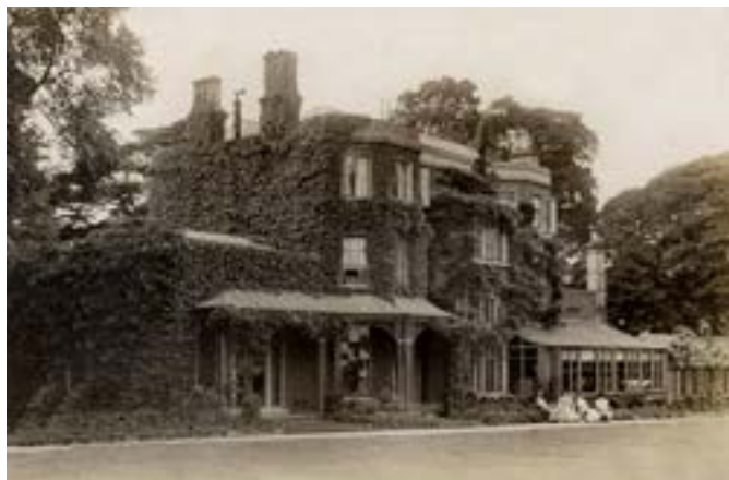
The house on Denmark Hill
