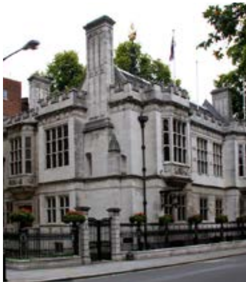
Two Temple Place on the Thames Embankment
