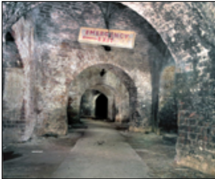
Railway Vaults at Camden
