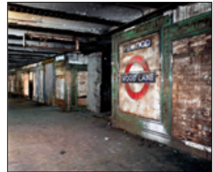
Wood Lane ghost station
