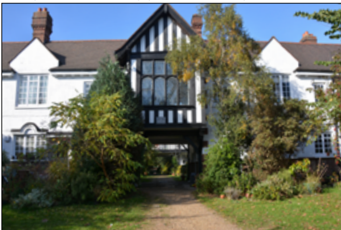
The Quadrangle at 34 Herne Hill also locally listed
